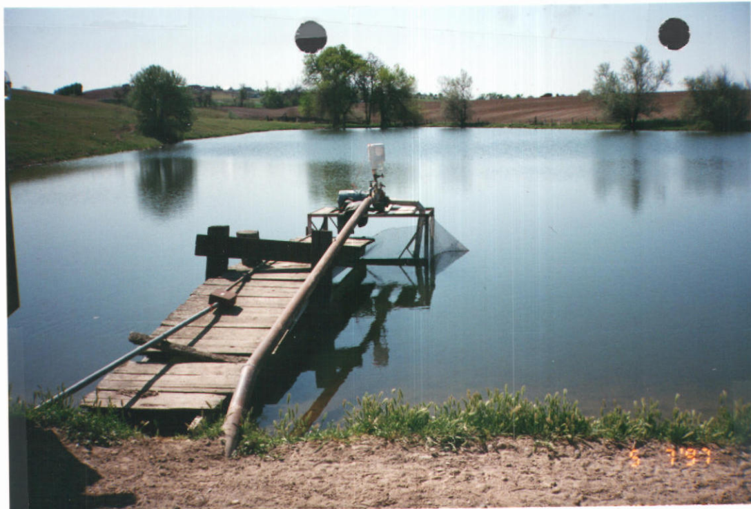
Pond & pump. View west east from dam
