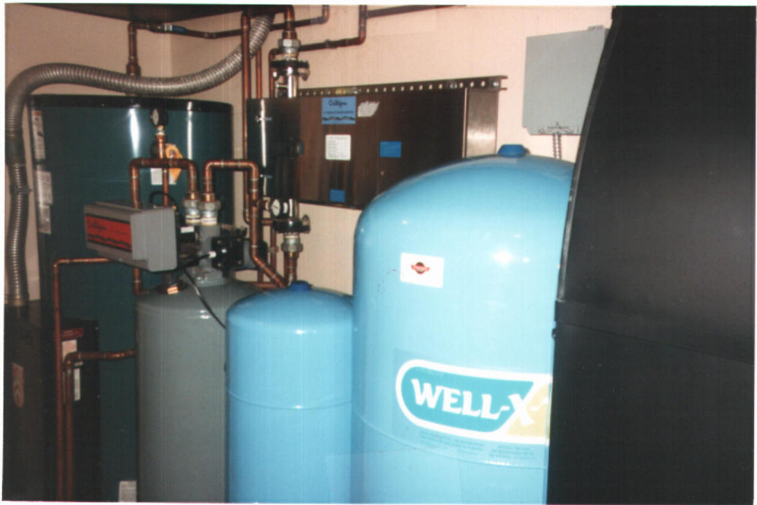
PHOTO TWO- Two pressure tanks, water heater, Culligan water conditioner and Culligan ultraviolet water purifier in garage of home.
