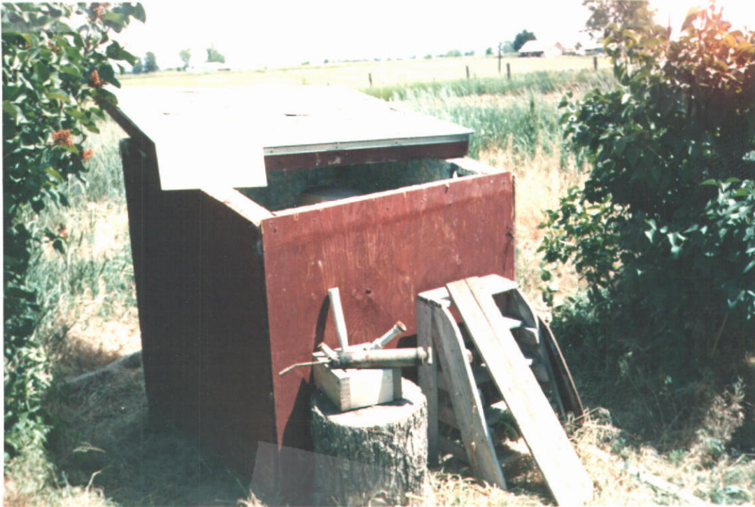
#1 View of wellhouse
