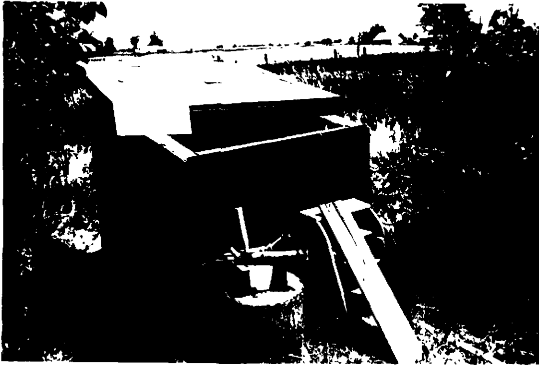
#1 View of wellhouse
