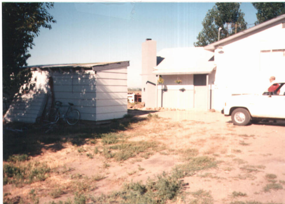
#2 View of shed where well is located.
