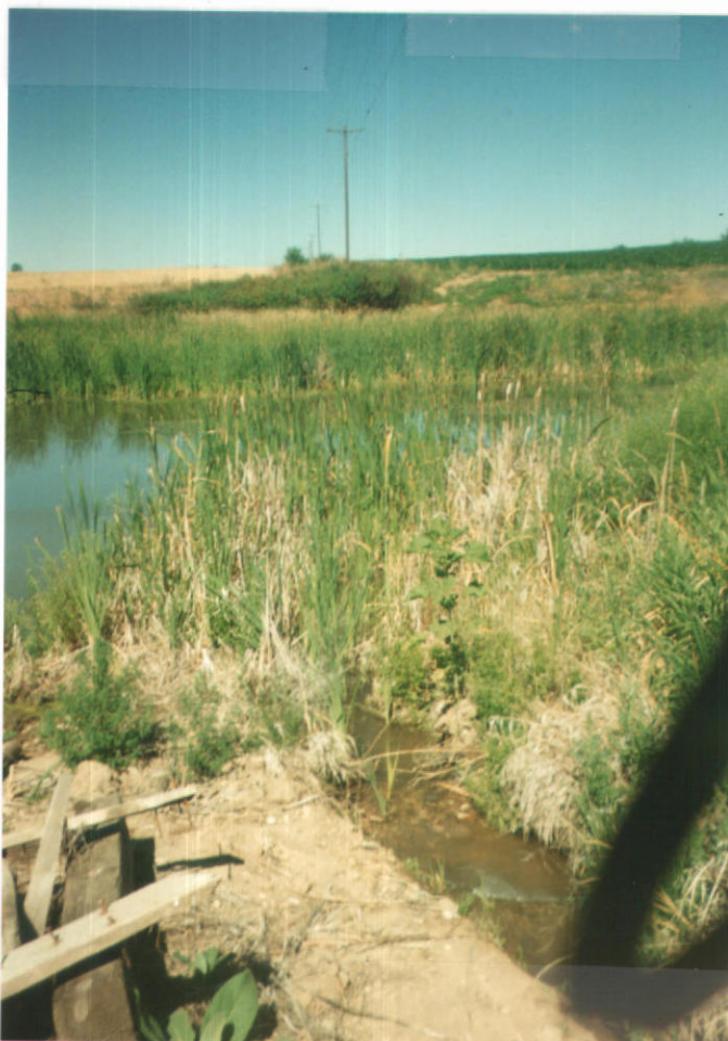
VIEW OF ONE OF THE TWO WASTE WATER INLETS.
