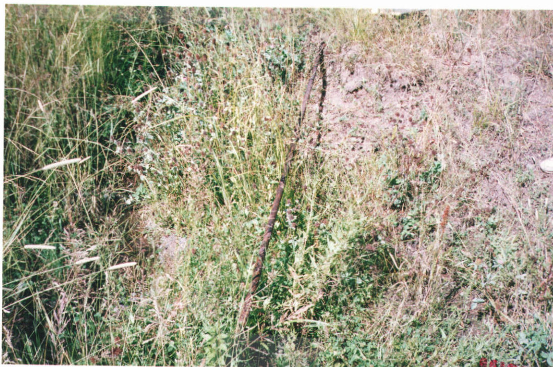
Service line, 3/4" Iron pipe, leading to home. JAN. 18 1994
