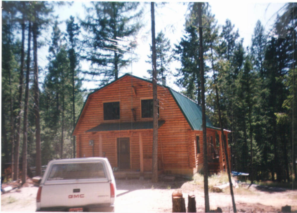
View of the Meidinger domestic. View is looking south. Some external use is visible on the south (other) side of the house.
