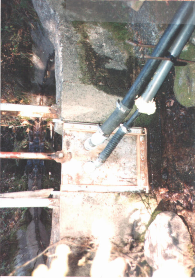
HAY CREEK DIVERSION DAM & GATE COMPLETE CLOSED. ALL WATER GOES THRU PIPES.
