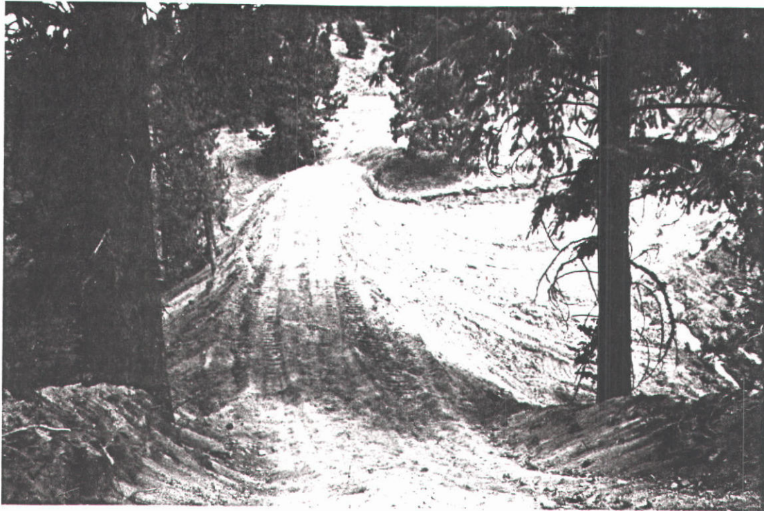
① Looking North at earth dam is 5\frac{1}{2} SE SW. Drainage flows to left in picture. (cuts #1 per logs)
