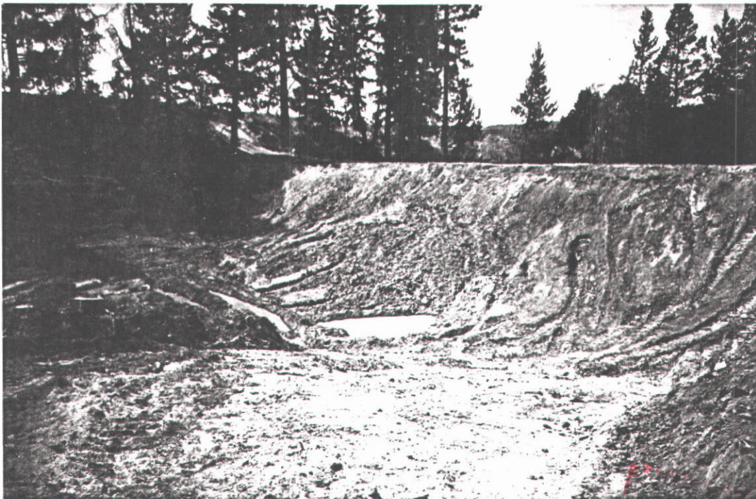
② Looking SW at back side of earth dam
