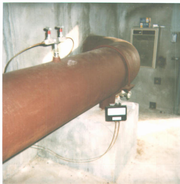
Diversion Penstock with Moter 65-13619 9/3/96
