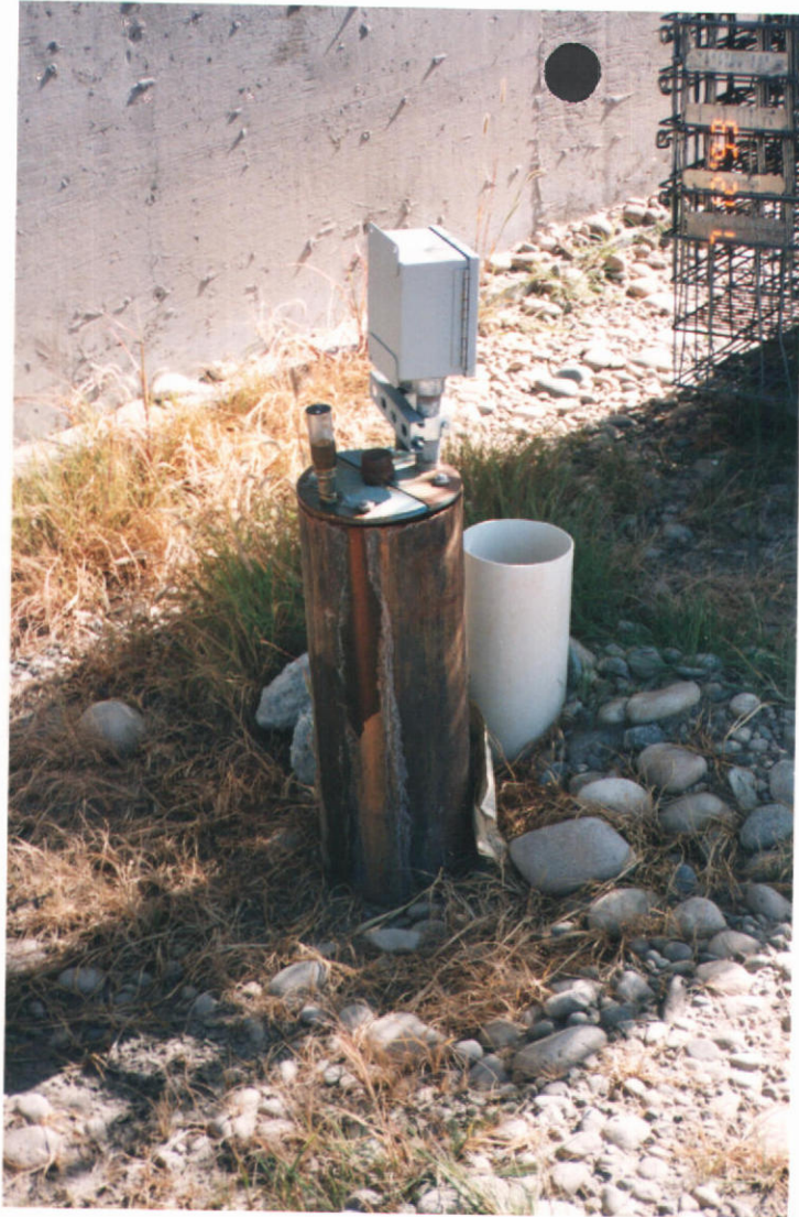
2 8" wells with 5 HP submersible pumps
