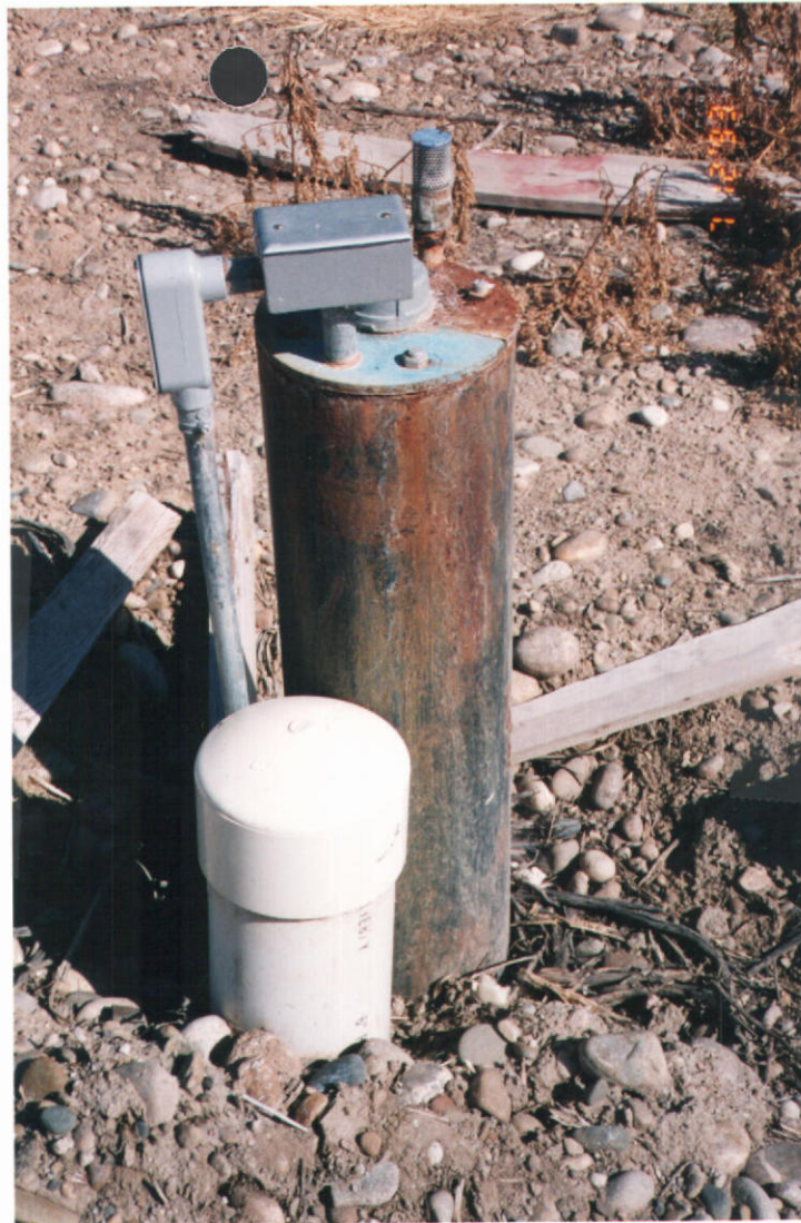
2 8" wells with 5 HP submersible pumps
