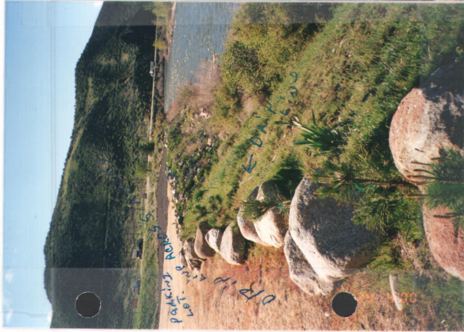
A Drip line Runs Along The Rocks Around Parking Lot
