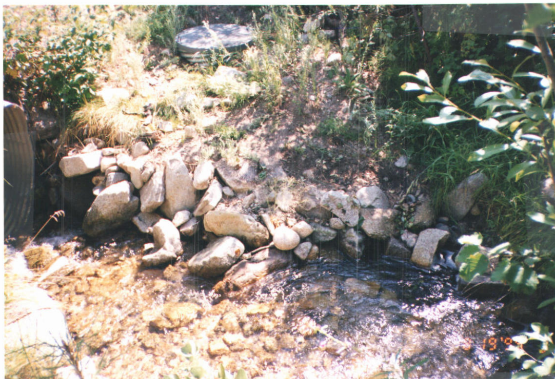
48" Cmp at Left; Seven Peaks Rd. Culvert
