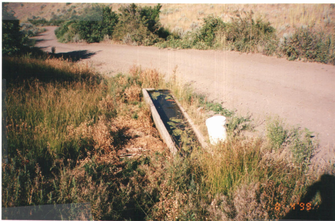
View Looking SW
