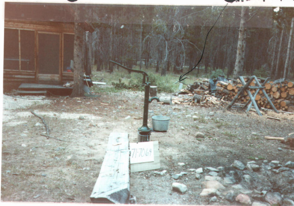
New well and hand pump
