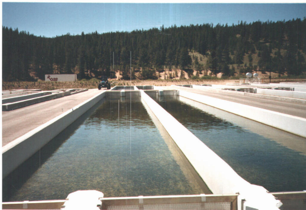
Large Raceways. Looking West
