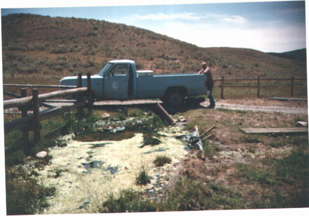
45° & Pipe discharges Into ditch System Here.
