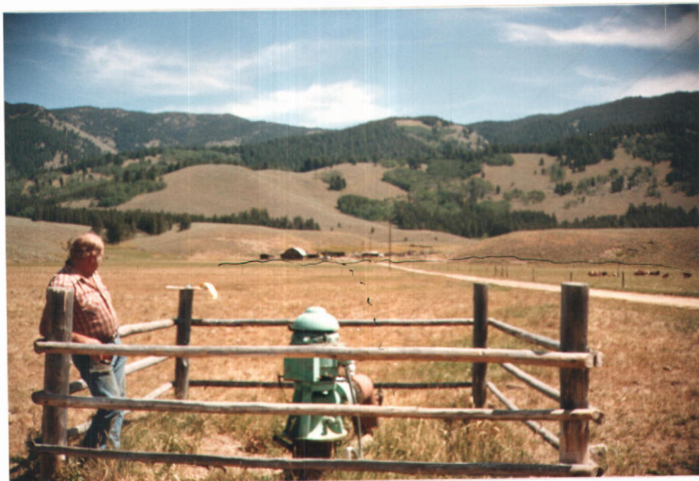
Looking Towards discharge point near Barn across Plu
