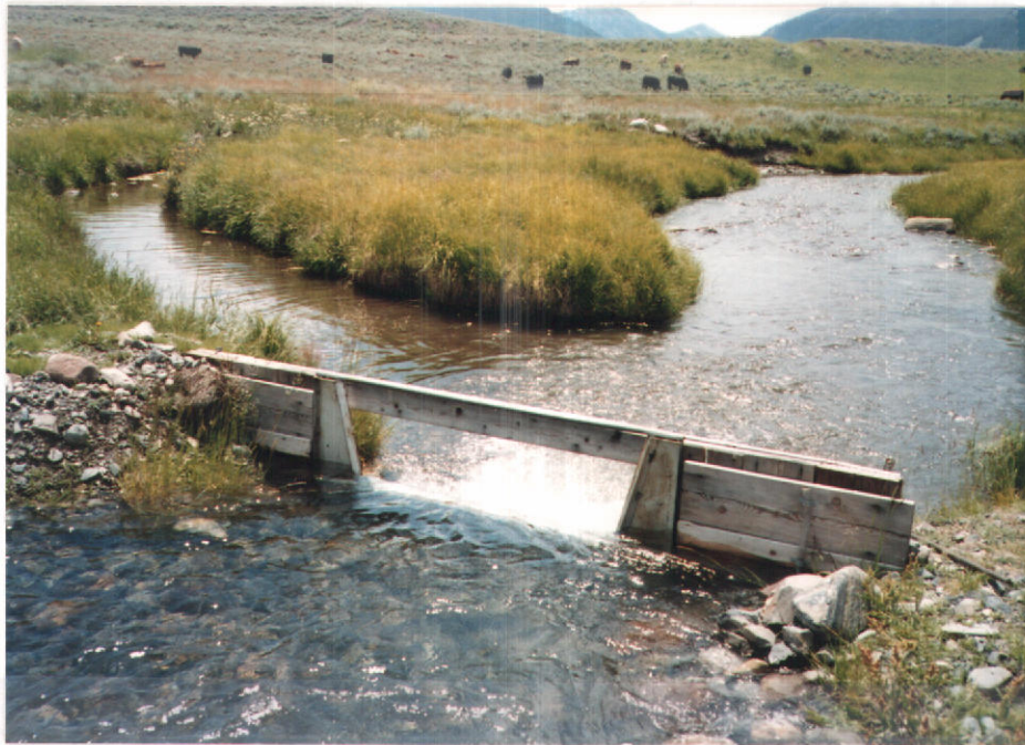
Return Flow to Pole Creek
