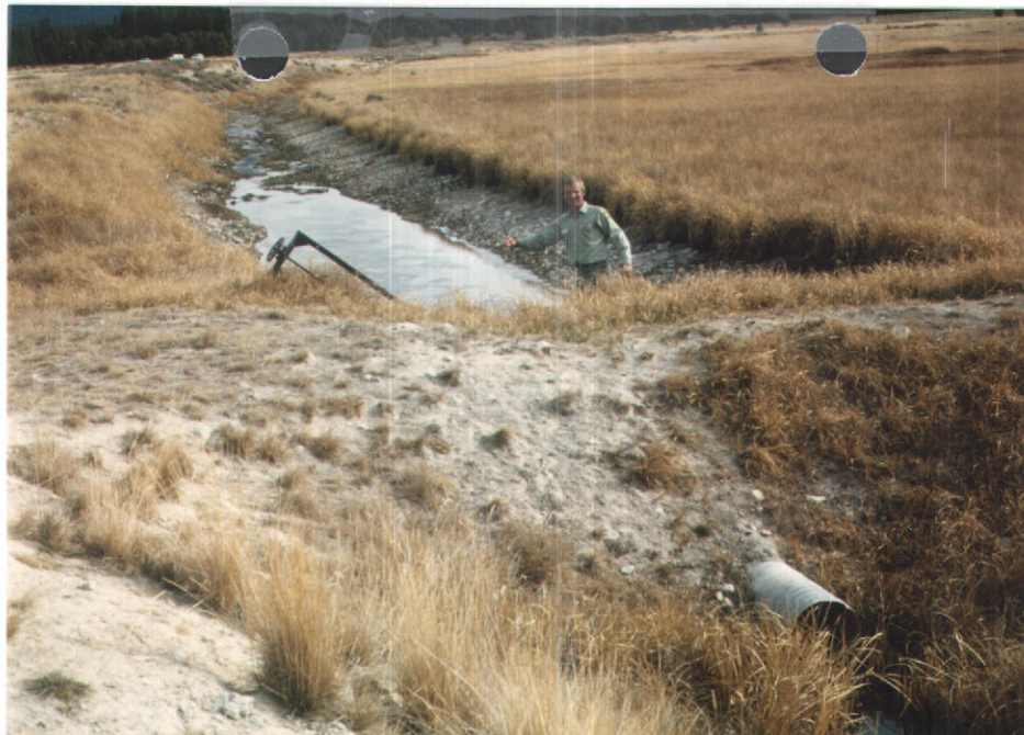
71-07122 DITCH WITH CULVERT AND VALVE BEING REPAIRED
