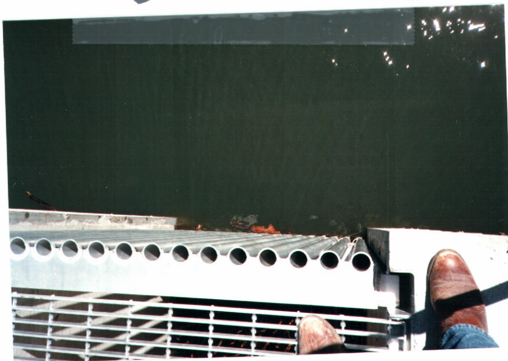
Screens on Inlet of Head Box
