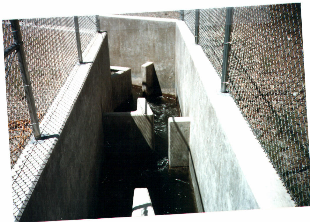
Fish Ladder at tail of Fish Trap
