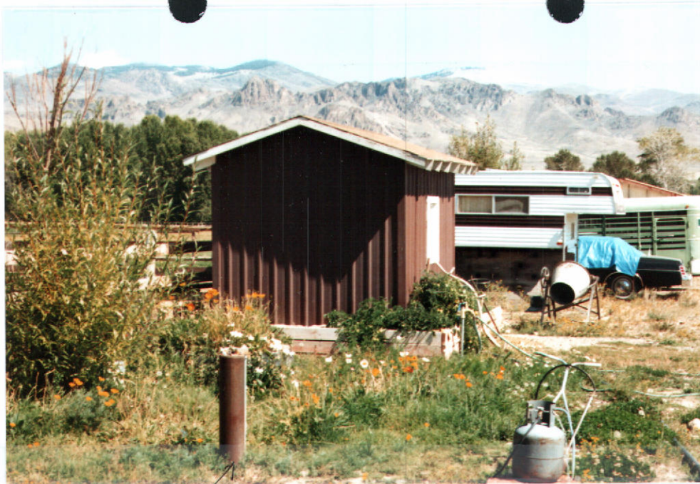
Point of diversion and well house
