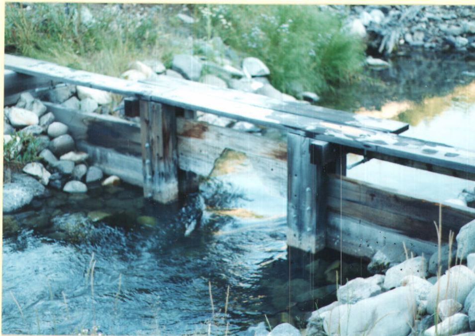
Pond Series No. 1 - Check Structure No. 2
