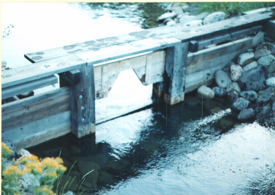
Pond Series No. 1 - Check Structure No. 3
