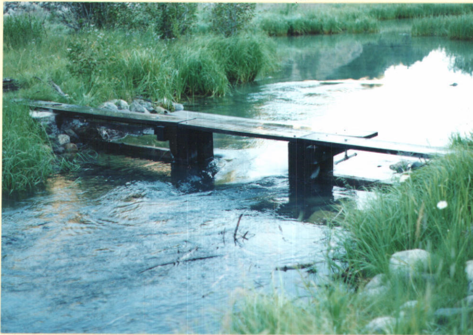
Pond Series No. 1 - Check Structure No. 1
