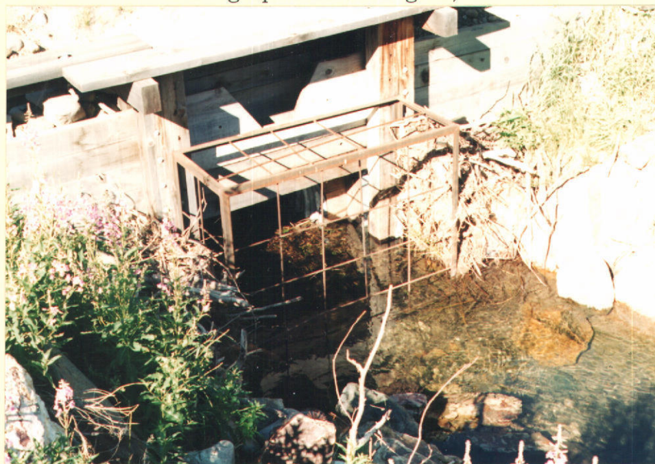
Pond Series No. 4 - Inlet Structure
