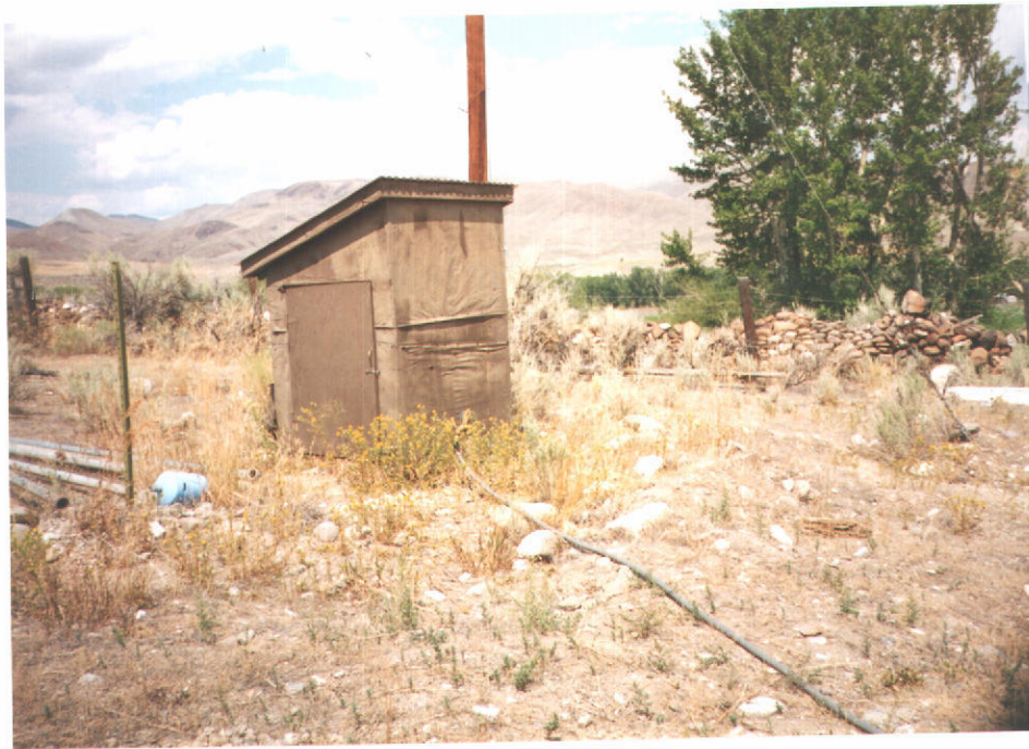
72-07502 WELL HOUSE WITH HYDRANT LOCATED AT THE END OF DRIVEWAY ON THE NORTHSIDE OF PROPERTY
