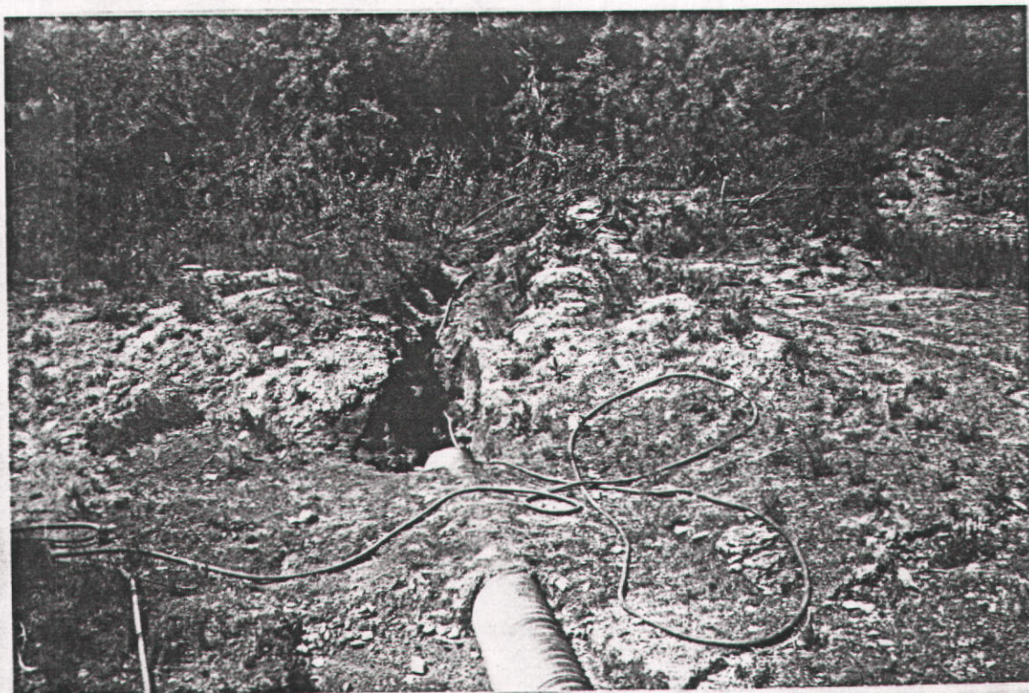
Picture No. 10 LOOKING UP- STREAM TO WHERE OVER- FLOW COMES OFF OF THE HILLSIDE AND DRAINS INTO CONCRETE PIPE
