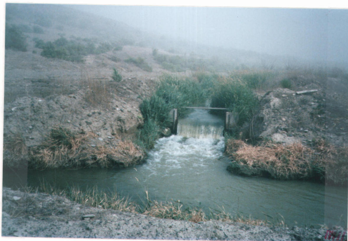
- Rectangular Weir Below Tate Reservoir -
