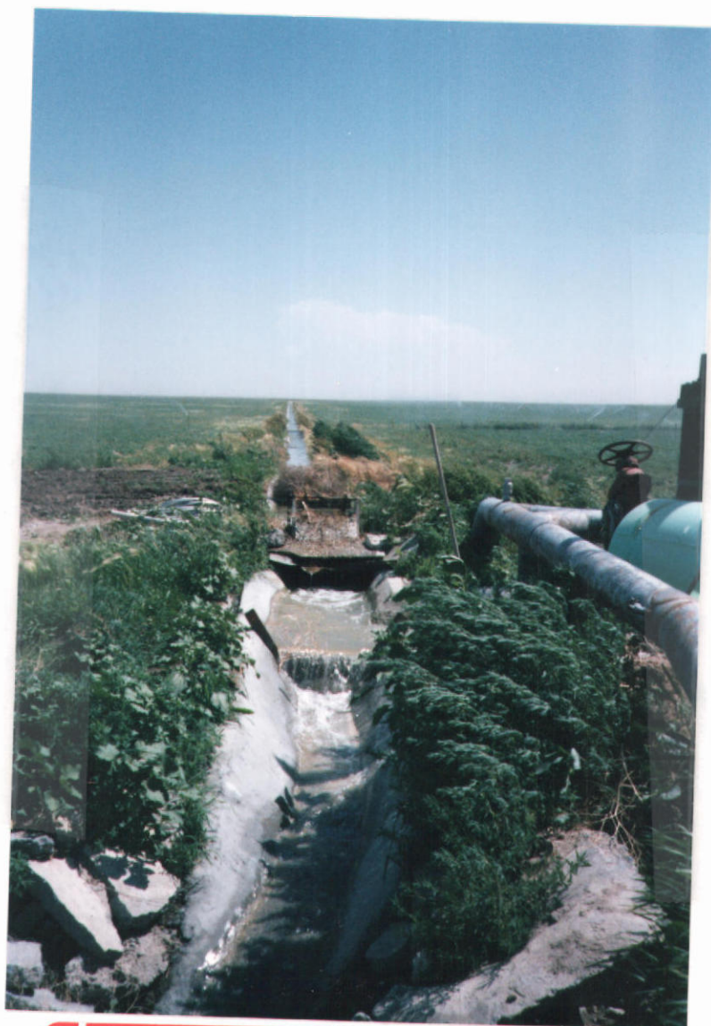
- Ditch to 100 HP Relift Pump -
