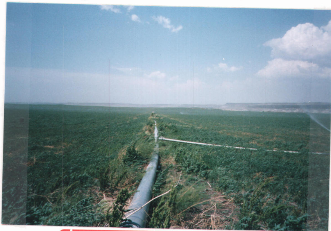
- Mainline from Bybee Reservoir -
