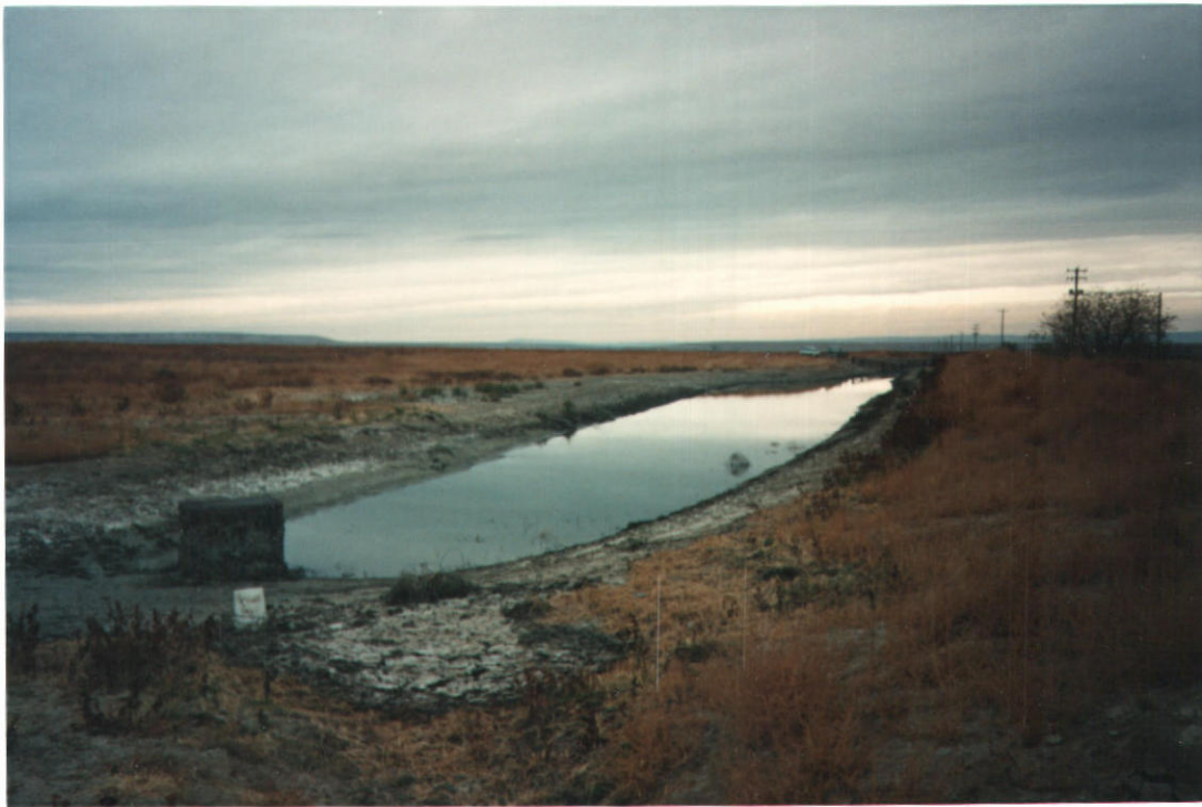
OUTLET OF RELIFT POND
