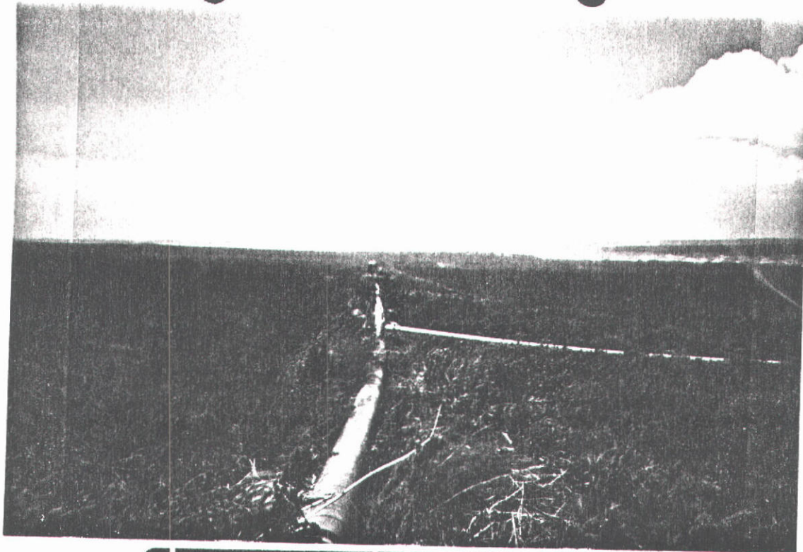
- Mainline from Bybee Reservoir -
