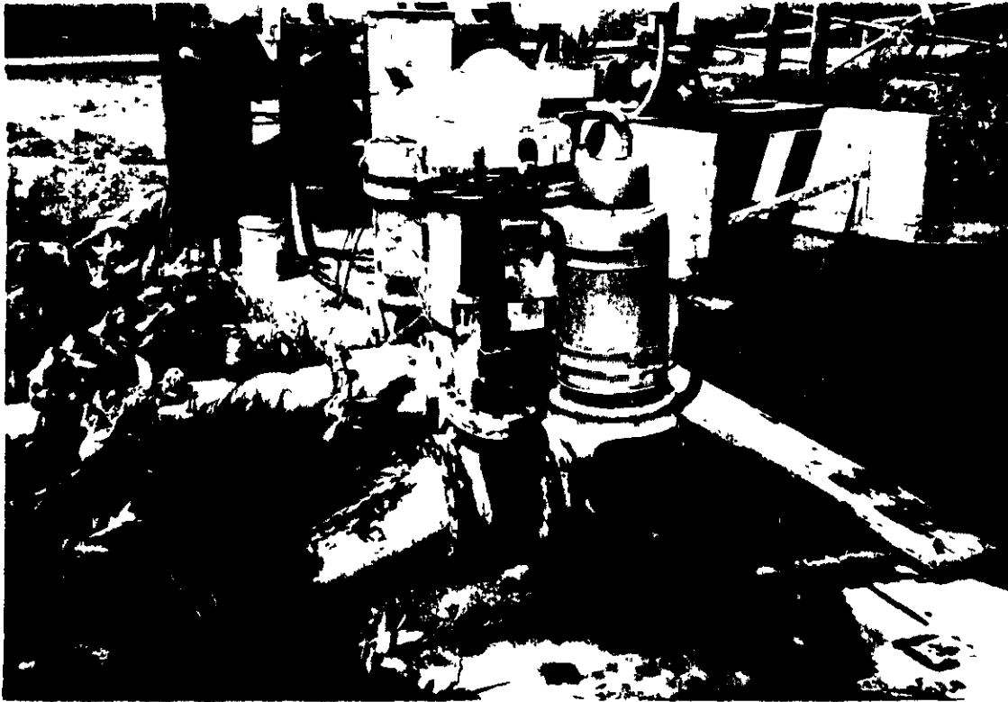
- 40 HP Pump at Bybee Reservoir -
