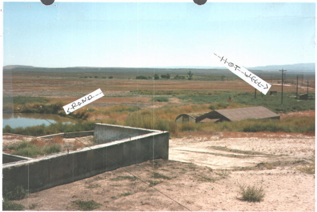
PICTURE # 1. LOOKING S.W. FROM BACK YARD. OVERLOOK SHOWING LOCATION OF POND AND HOT WELL.
