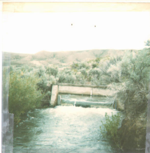
Looking upstream at the 10 foot long cippoletti weir measuring flow from discharge tunnel to Murphy Mutual Canal
