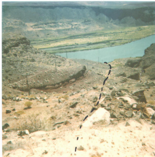
Looking towards Snake River down route of pipe line feeding Murphy Flat Canal. P12
