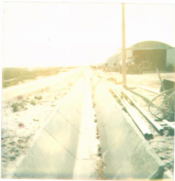
Looking east down lateral which carries water from Murphy Mutual Canal to Ponds 3 and 4. p9
