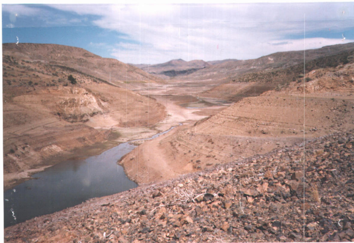
Looking Northeast at the reservoir area from the top and center of the dam.
