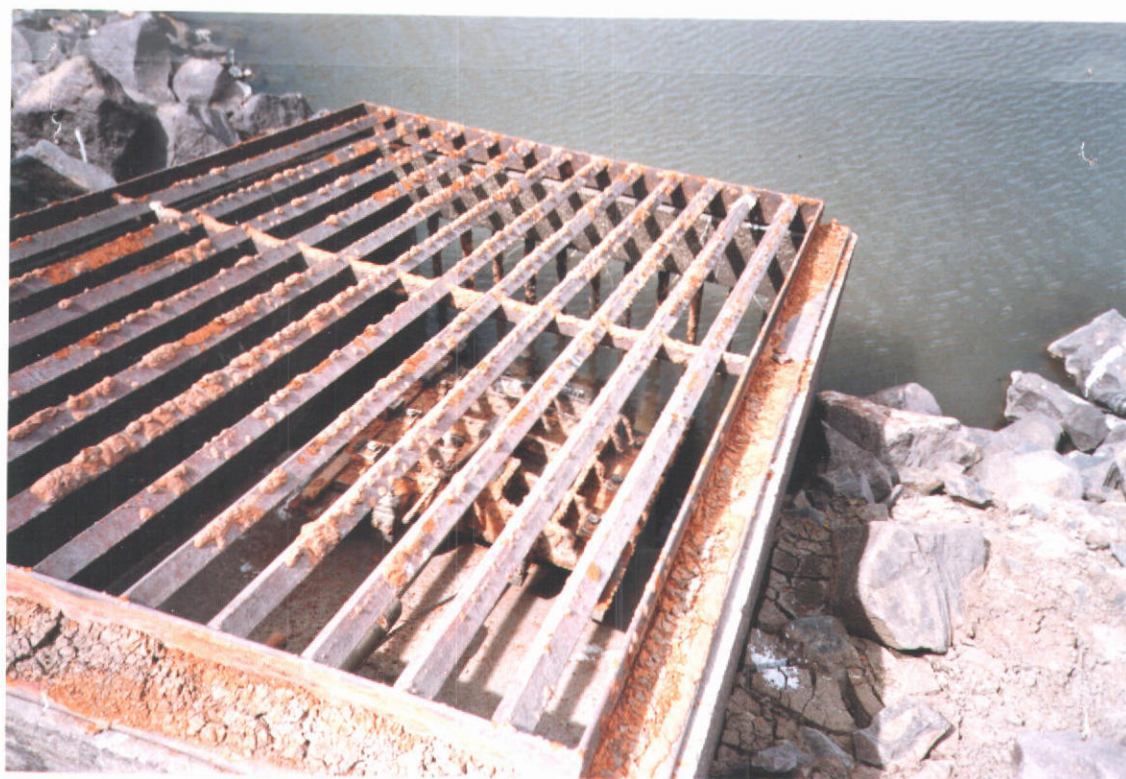
Facing looking North and down looking down at the control gate
