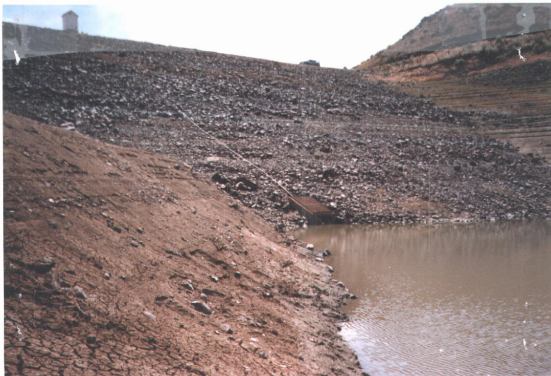
Looking South west at the control gate
