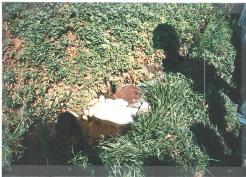
Springs #2 can only be seen by the overflow outlet, pipeline and ditch which run parallel to the Snake River to the house and stock.
