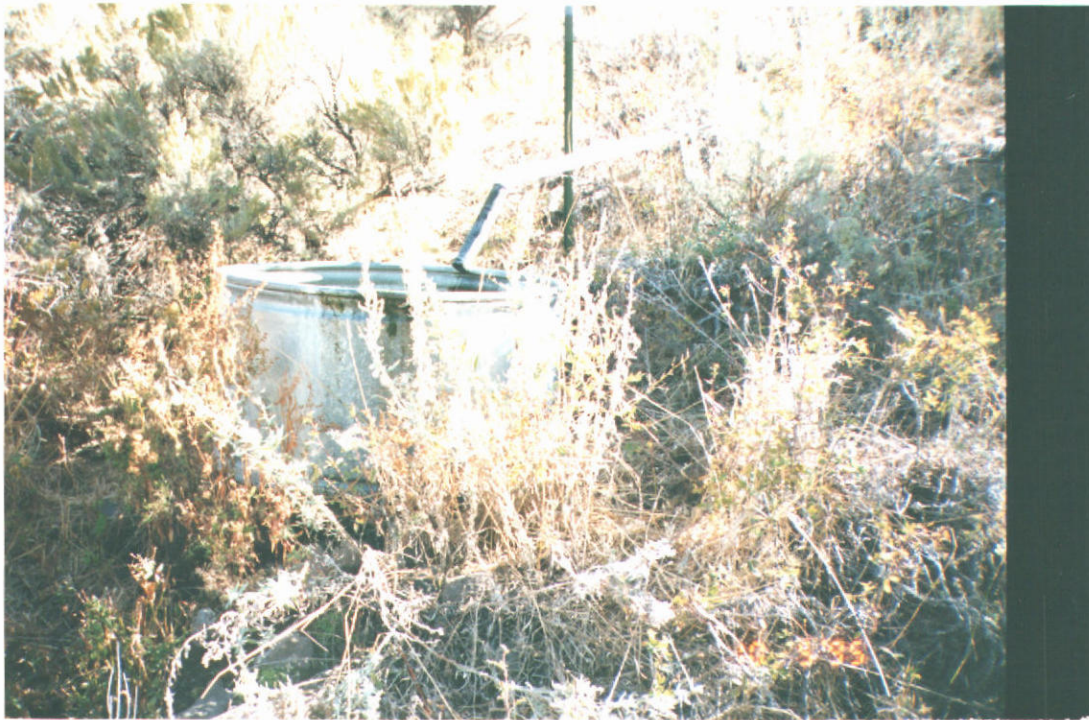
Stock tank #1 pipeline comes down from collection
