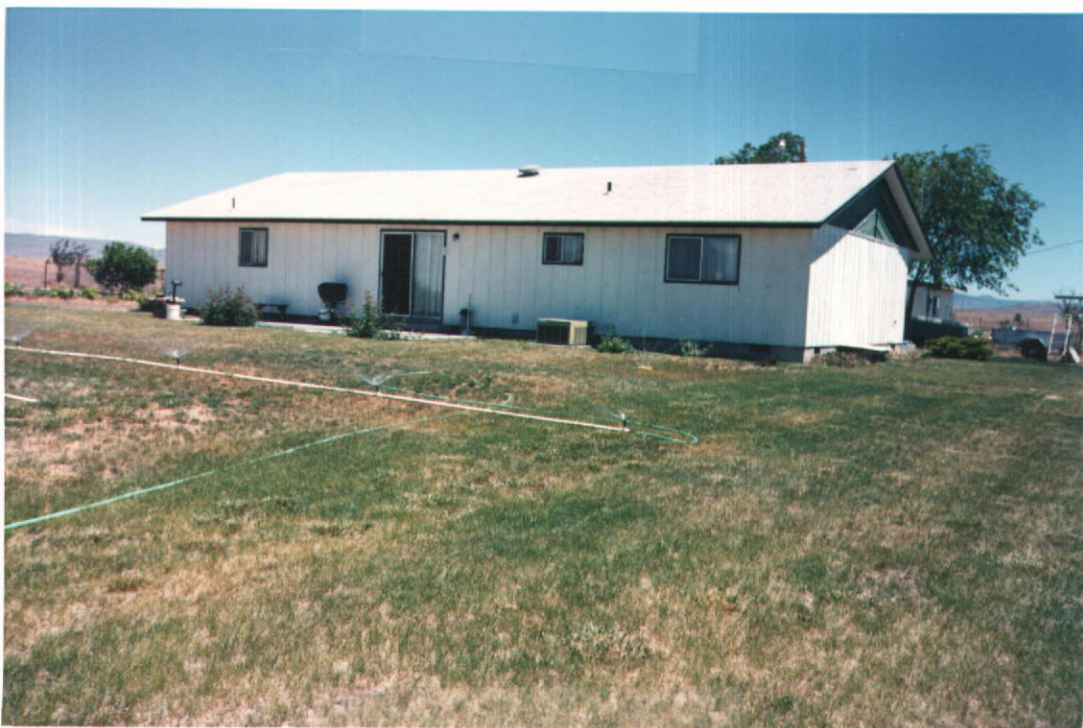
DOMESTIC + LAWN FACING NE
