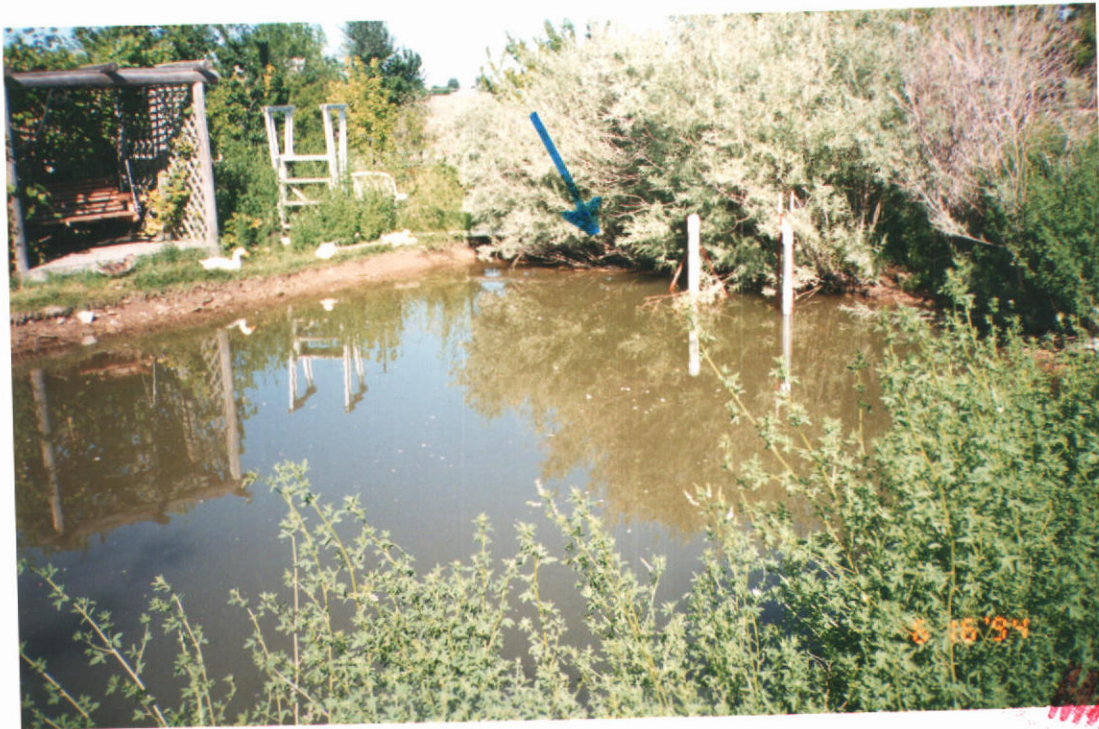
Pump station is just out of lower photo to ← the right
