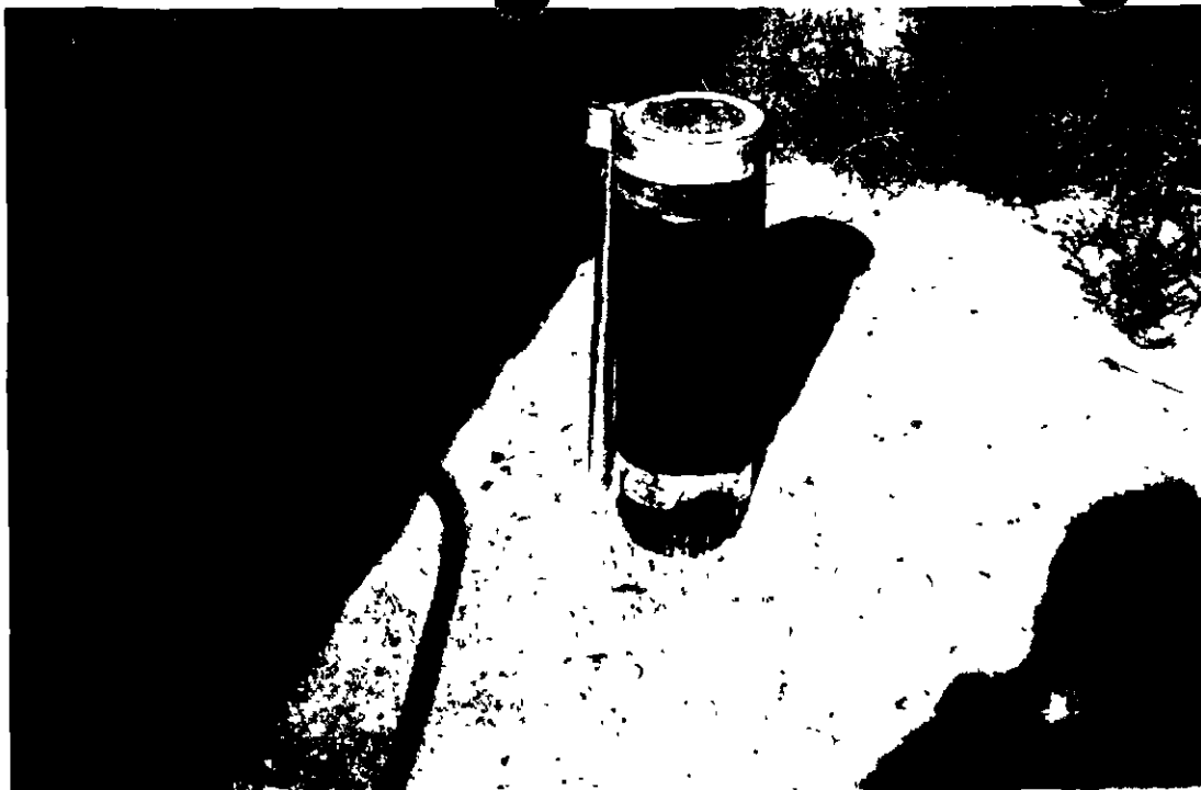
6" well 2.5 HP sub- mersible pump
