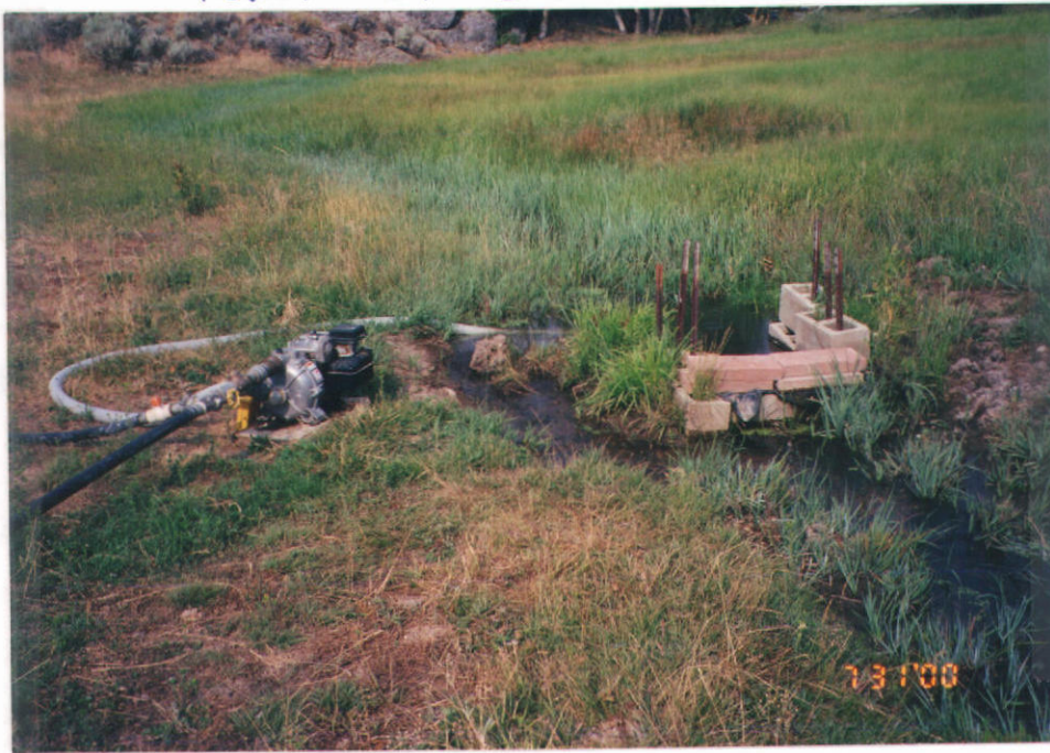
Point of Diversion
