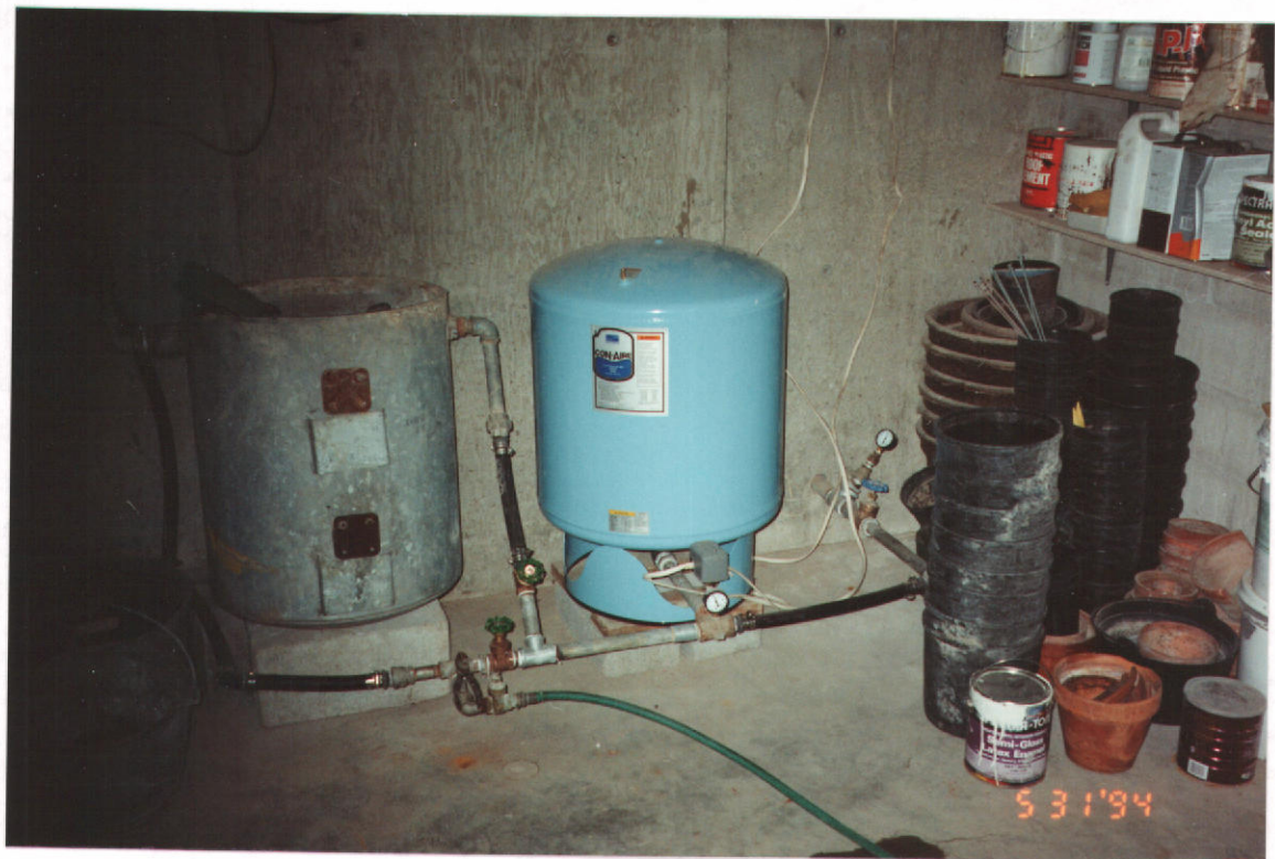
PRESSURE TANK SYSTEM IN BASEMENT
