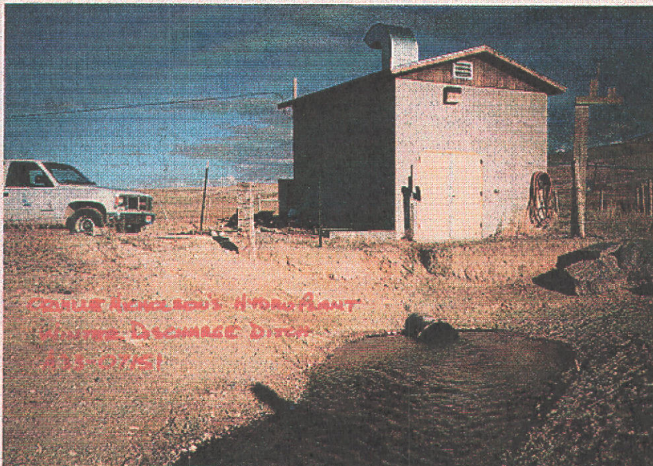
Photo 5: WINTER DISCHARGE FROM TURBINE
