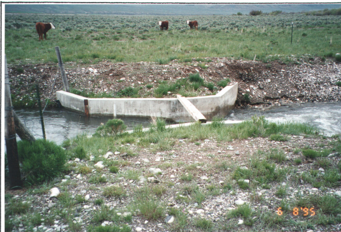
FLUME POINT OF RETURN DISCHARGE TO WET CK.
