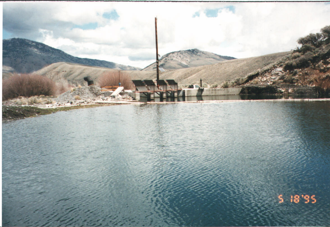
VIEW OF HYDRO SYSTEM INTAKE AT DRY CREEK RESERVOIR
