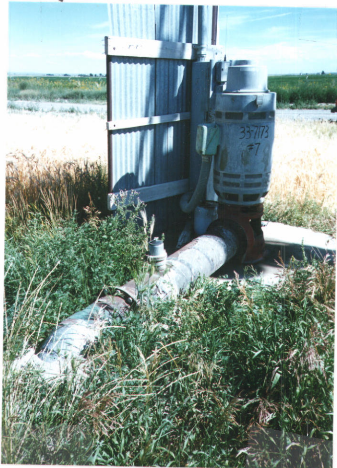
↙ VIEW TO SOUTH
