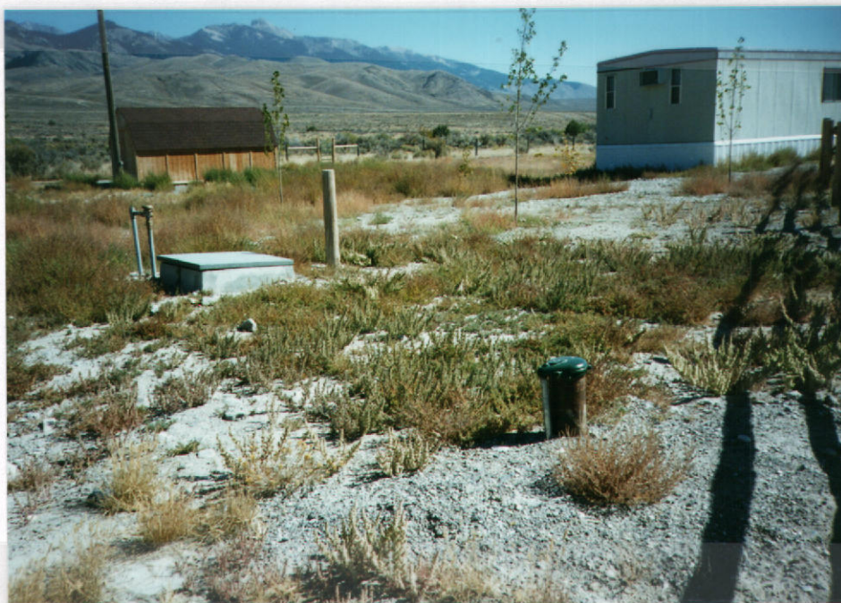
Fig. 2 - Point of diversion showing vault.
