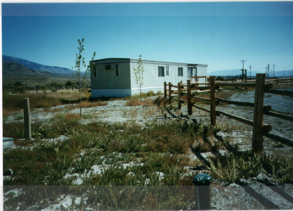
Fig. 1 - Point of diversion showing domestic place of use.
