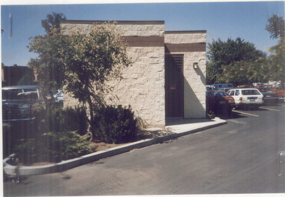
P.D. The production well pump station. Looking North- west
