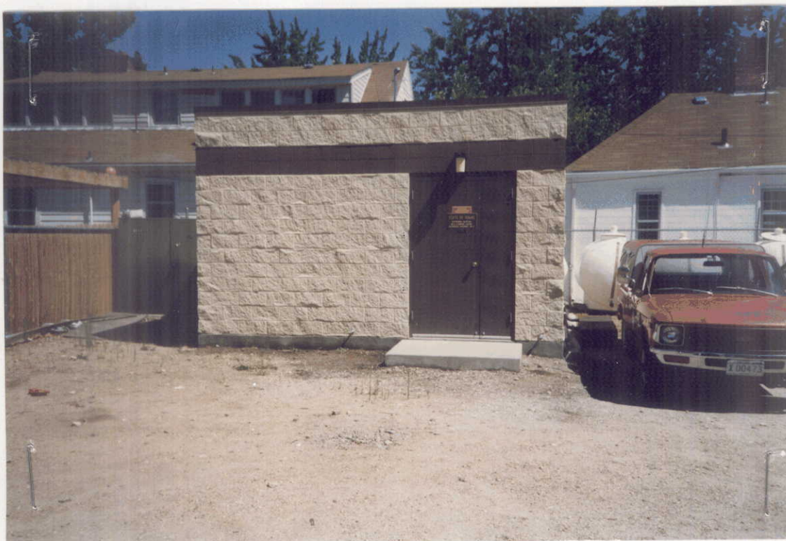
The injection well pump station, Looking East.
