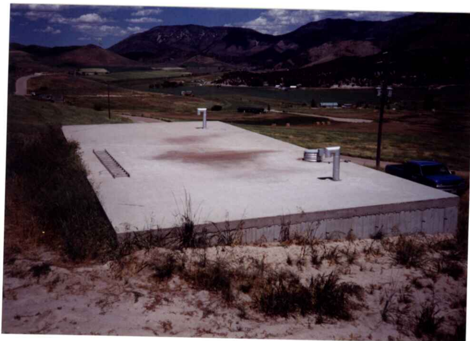
Looking North at top of tank
