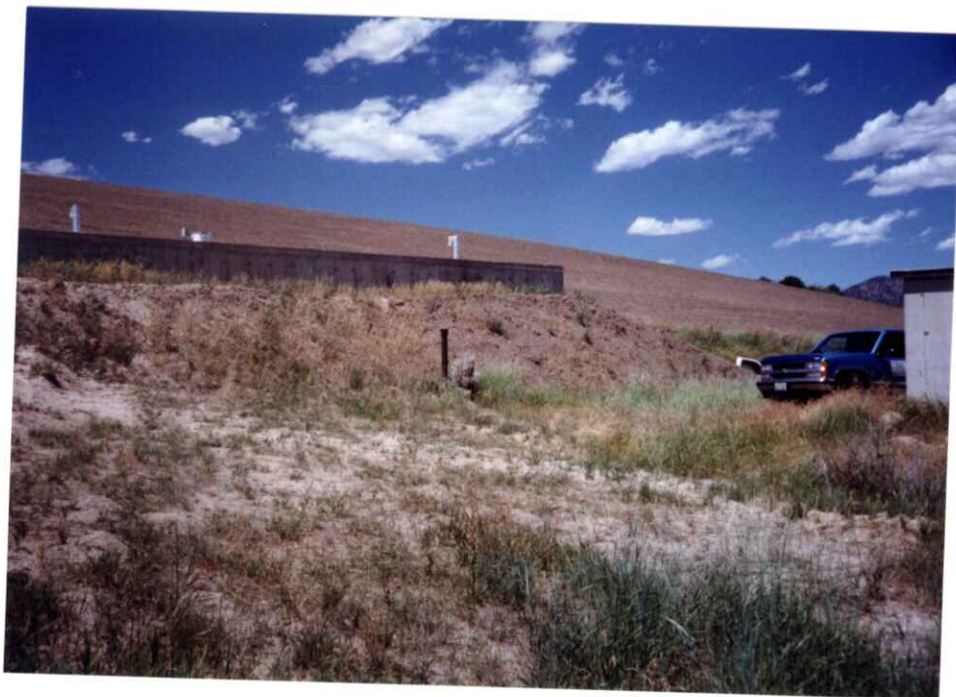
looking West at Tank
