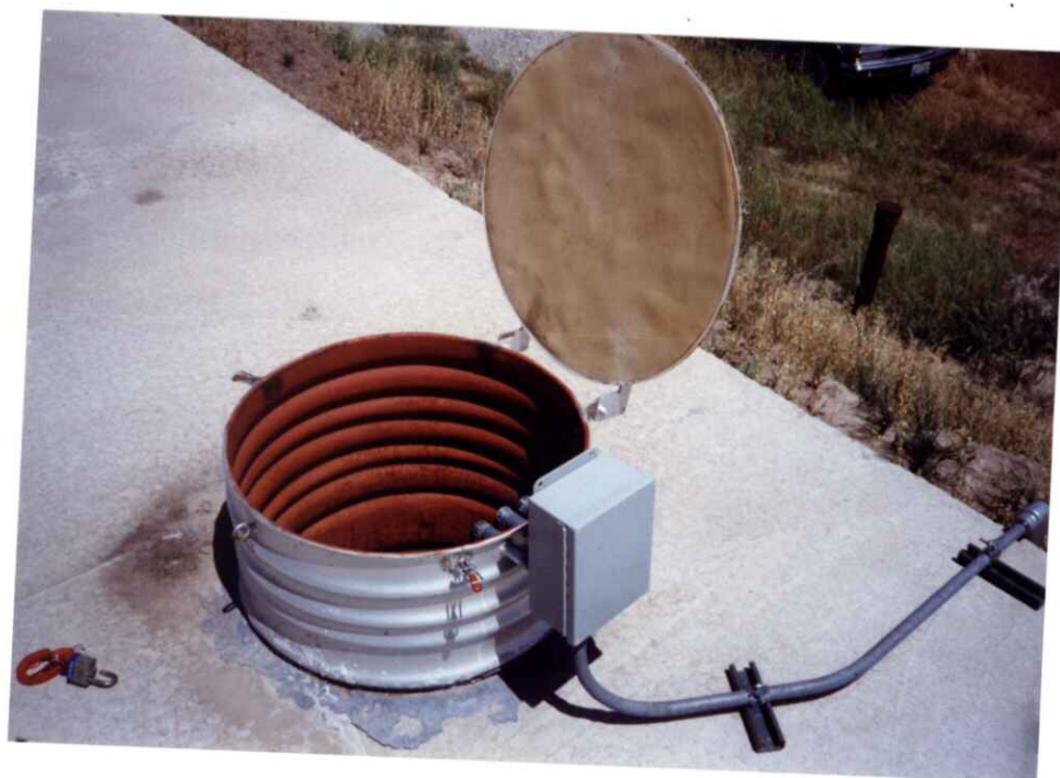
Entrance to Tank,
