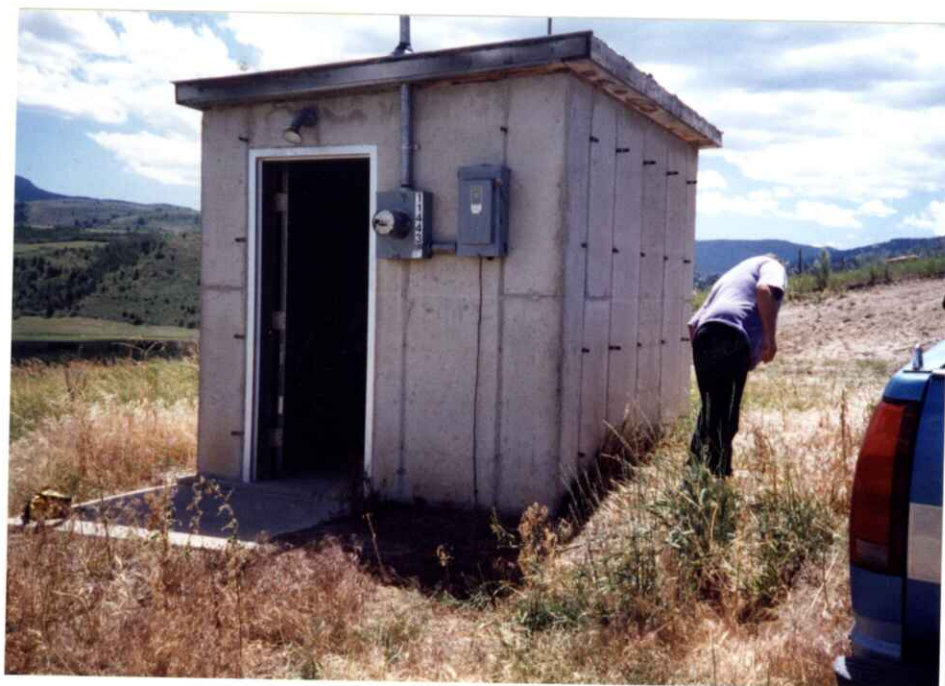
Looking South at well house
