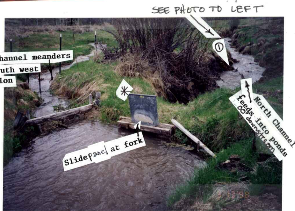
Slide panel at fork PHOTO LOOKING SW'LY ±
