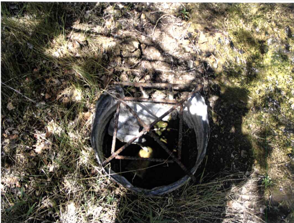
Overflow structure directly adjacent to channel #1 just upstream of falls to pond #1. Pipe in structure to unknown location.
