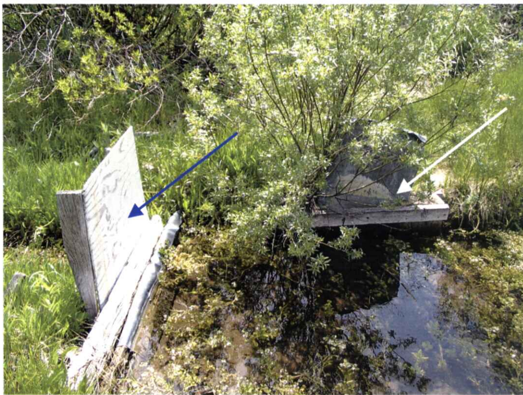
PoD. White arrow into channel 1. 95% of (very low) flow was being diverted this direction on June 16, 2005. Blue arrow into channel #2. A small amount of water was getting into channel #2 – probably not on purpose, dam is sort of leaky.
