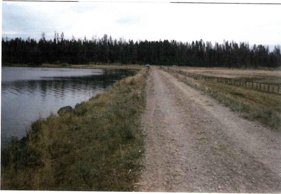
CREST OF DAM.
