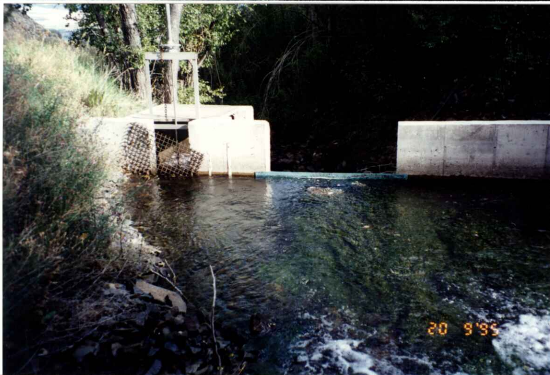
CITY OF SALMON MUNICIPAL WATER INTAKE ON LEFT. POINT OF DIVERSION
