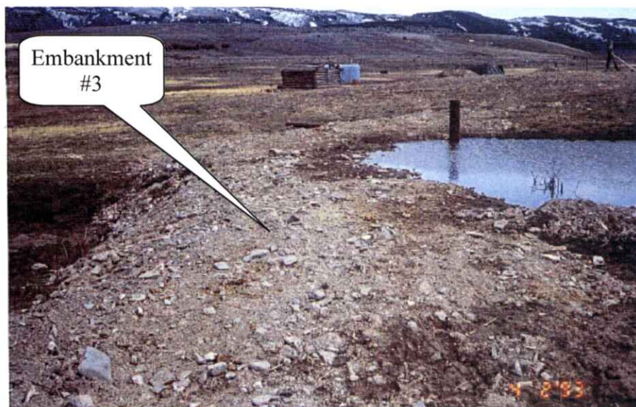
BELOW: View showing "Embankment #3". Photo, taken on April 2, 1993, was copied from Smyer West Dam IDWR Dam Safety File (D45-7608).
