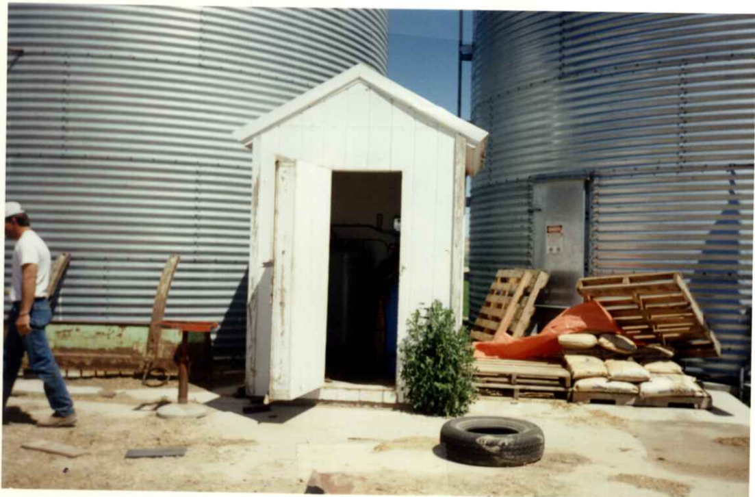
PHOTO TWO- Pump house located east of well. 6/13/06 Back-up well located inside pump house per owner
