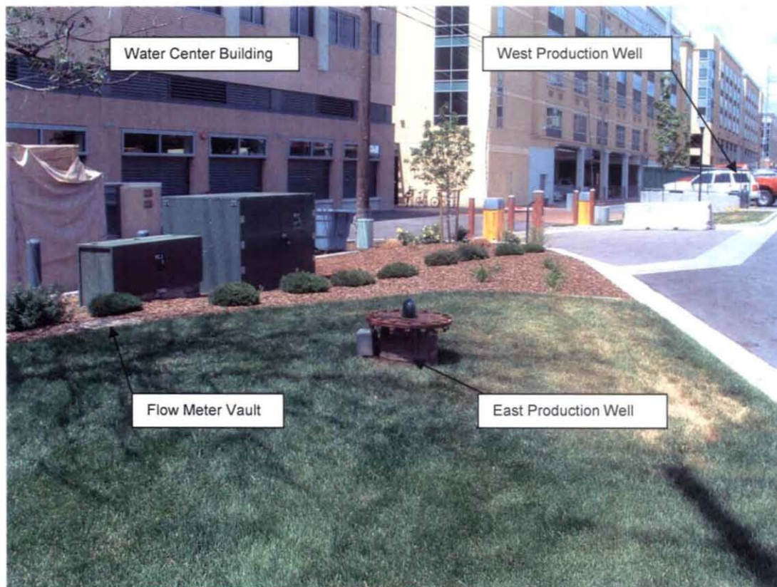
Figure 1. View of production wells on north side of Water Center.
