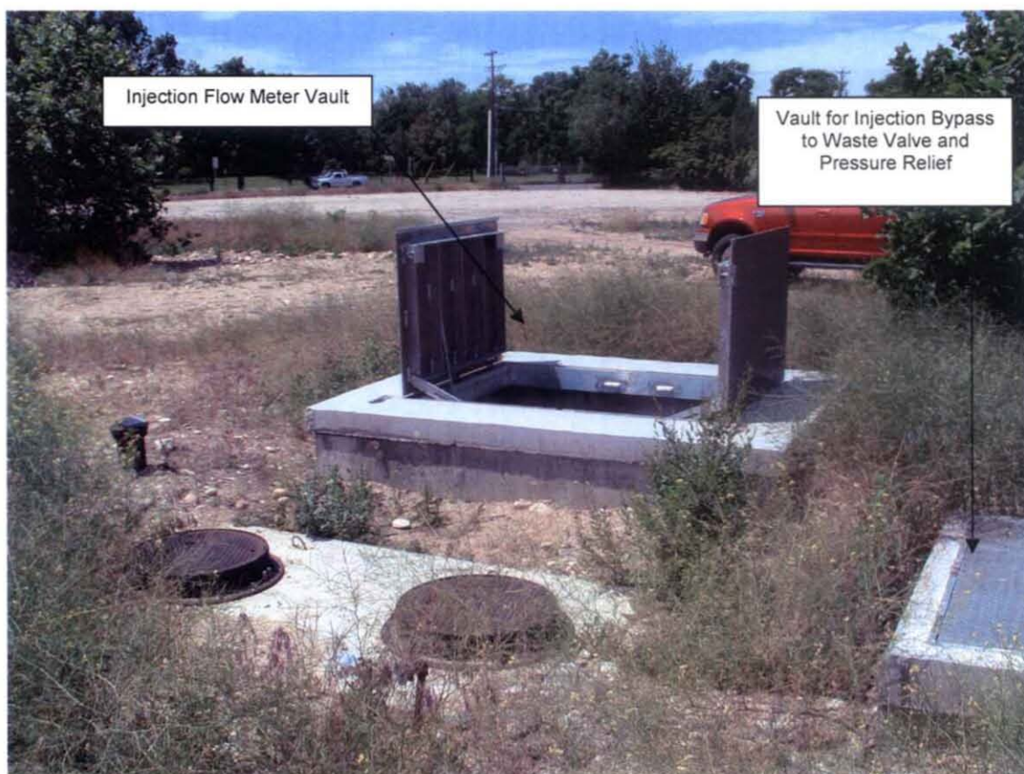
Figure 11. Injection well meter vault area.
